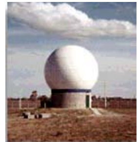
ORBCOMM Earth Station
