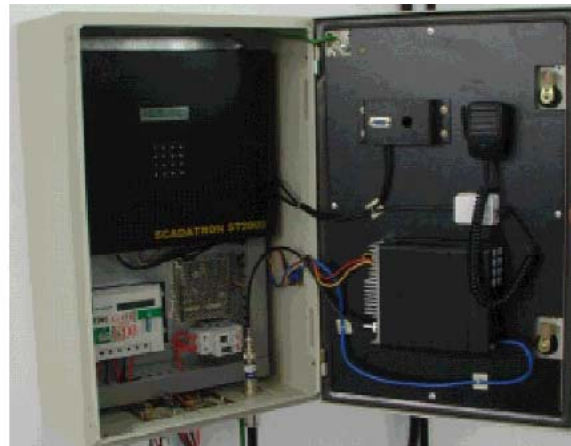
RTU with a wall mounting IP65 chassis
